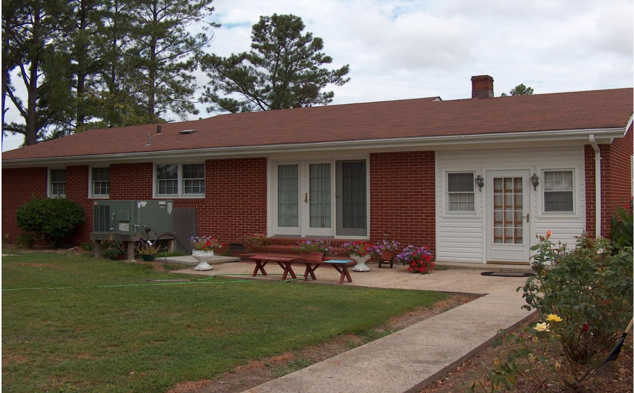
Photograph 2. Gloucester County Mitigation Project - Rowe House before Mitigation
