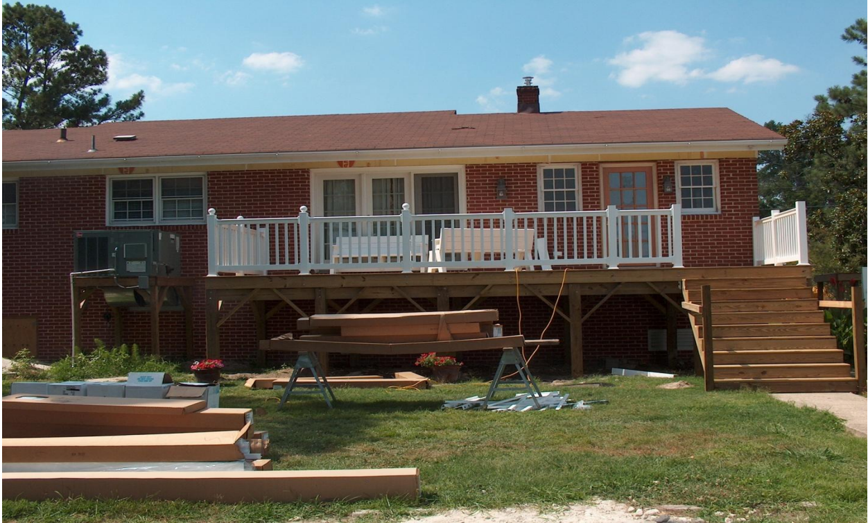
Photograph 3. Gloucester County Mitigation Project - Rowe House after Mitigation
