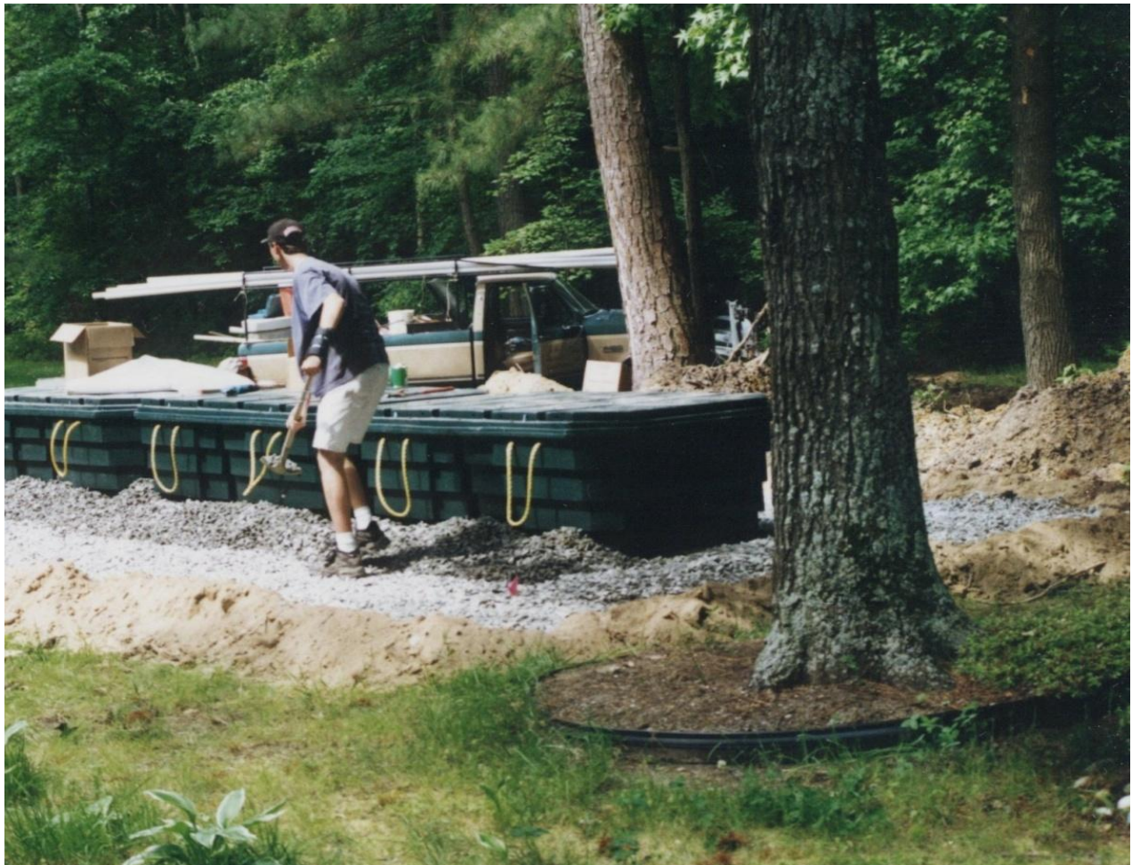
Photograph 1. Worker installing Puraflo System in the Middle Peninsula
