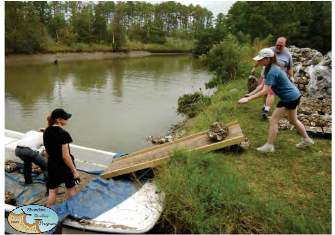
Lack of access at the site of placement meant that the bags had to be transported by boat. Because a 5 ft bank occurred at the staging area, a wooden ramp was built so the bags could slide down.
