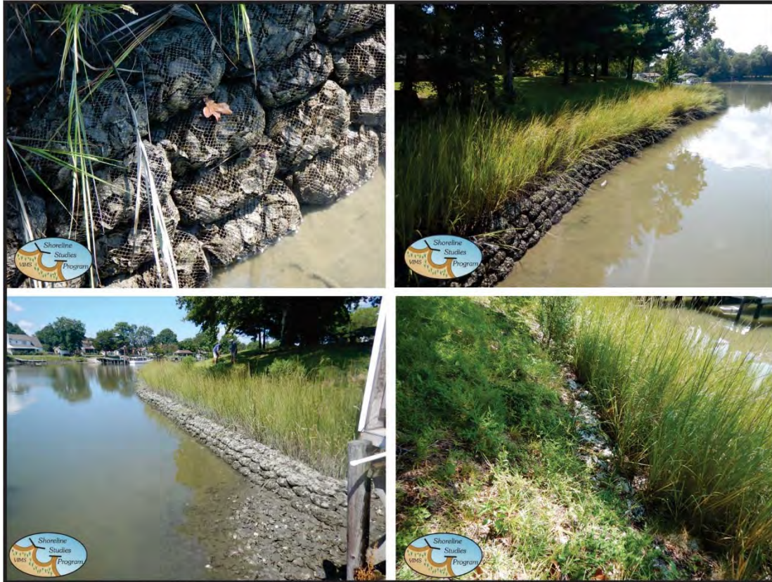
Figure 4-19. Site 4 oyster bag sill in September 2018.
