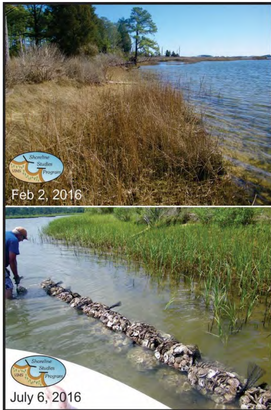
Figure 4-25. Site 6 Top: prior to installation, the site had an eroding marsh. Bottom: a 3-bag oyster bag sill was installed in July 2016.
