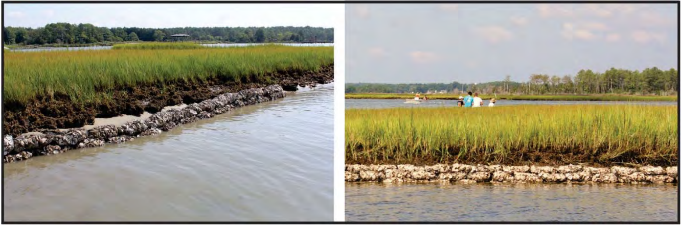
Figure 5-7. Construction of the 3-bag sill (left) and 6-bag sill (right). Photo credit: Linda Tjossem.
