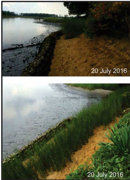
Figure 4-23. Site 5 during construction. Top: Sand was placed along the shoreline. Bottom: Marsh grass was planted. Photo credit: VMRC permit application.
