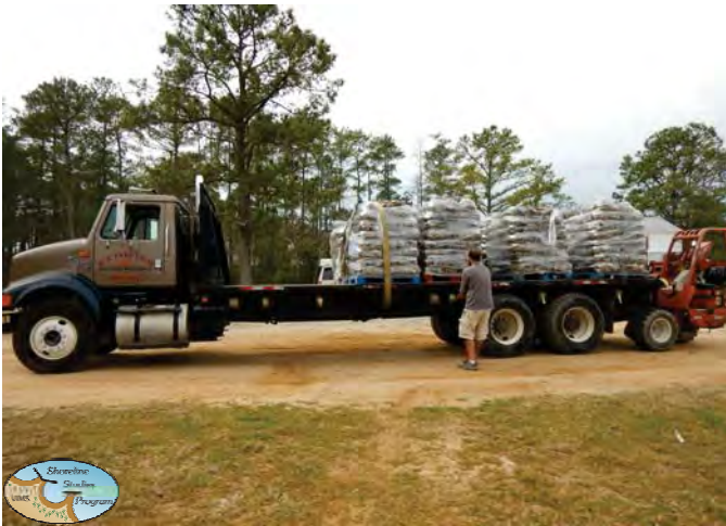
Oyster bag sills were delivered to the site by truck on pallets.
