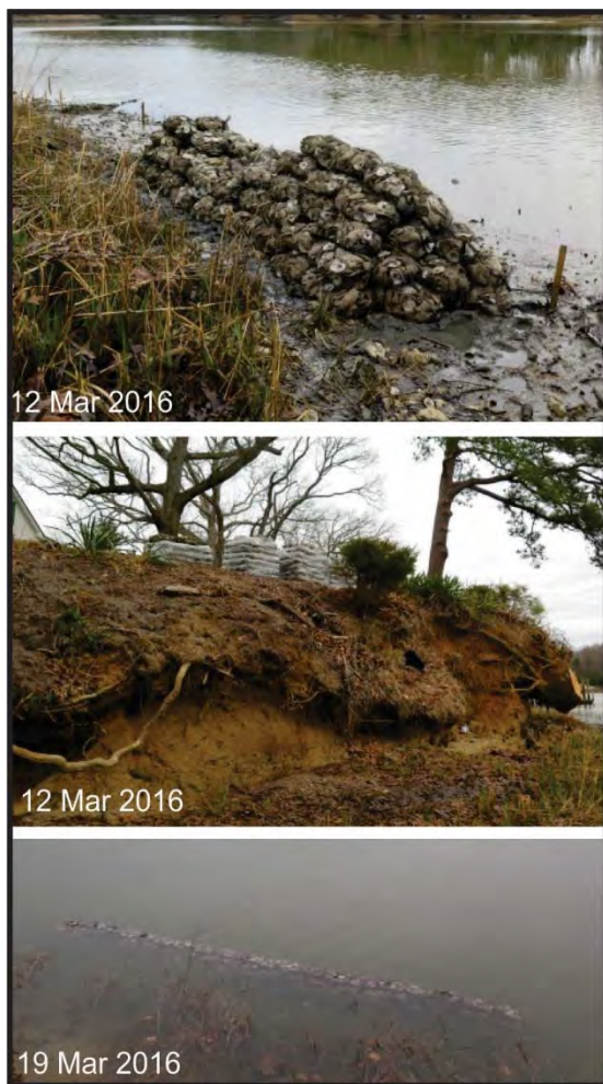
Figure 4-21. Site 5 during construction. Top: the bags are stacked in a 15 bag triangle at low water. Middle: the eroding upland bank was not graded. Bottom: the sill under high water. Photo credit: VMRC permit application.
