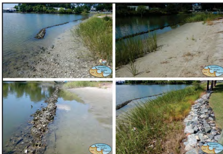
Figure 4-6. Present condition of Site 1 oyster bag sill (6 September 2018).
