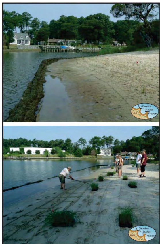
Figure 4-5. Post bag and sand installation at Site 1. The sand fill is visible landward of the sill, and volunteers planted grasses on the fill. Photo credit: Walter Priest, 29 June 2011.
