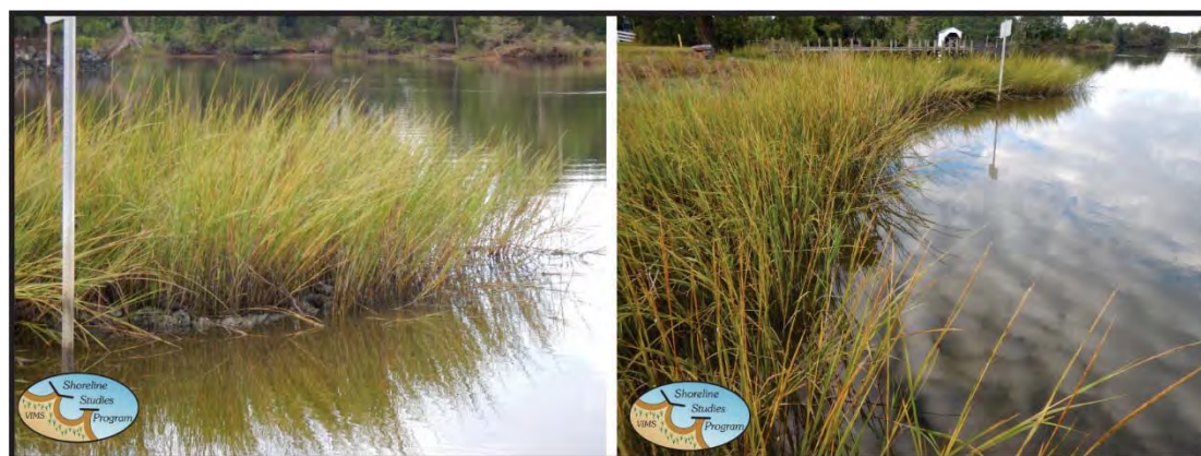
Figure 4-15. Oyster bag sill at Site 3, St. Johns Point in September 2018 approximately 4 years after placement.
