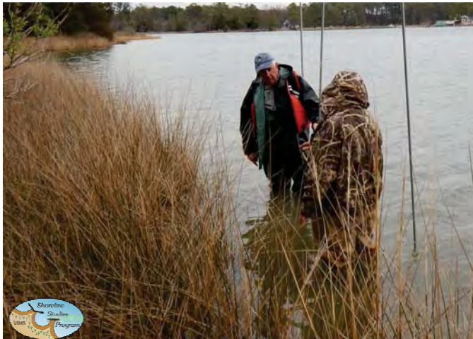
Metal pipe was installed to lay out the locations for the sills.
