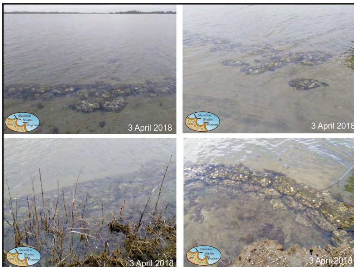
Figure 5-9. The three bag sill (top) that was placed on the southwest-facing shoreline has not been as stable. The top bag of some sections were rolled toward the shoreline. The six bag sill (bottom) on the point and the southeast-facing shoreline has remained intact.
