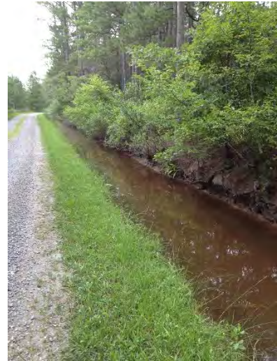
Photo 1 - Route 645 Roadside Ditch
