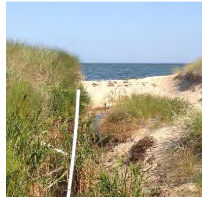
Photo 6 - Existing N. Bay Haven Rd. Outfall at Bay
