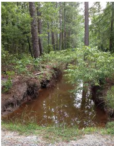
Photo 2 - Route 645 Outfall Ditch
