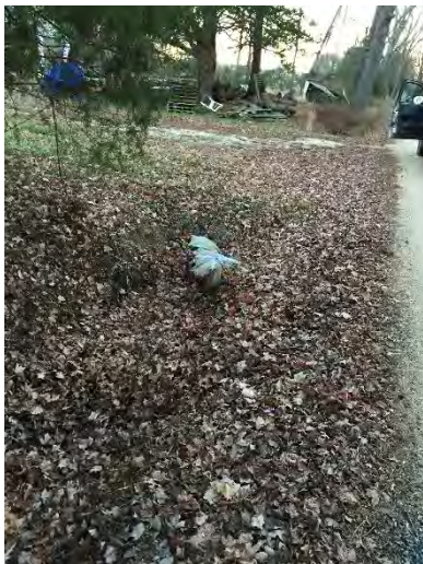
Photo 4 - Collapsed Culvert Along Peachie Lane
