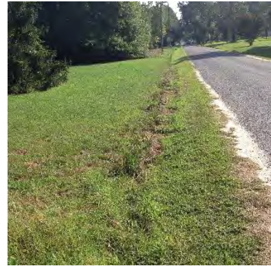
Photo 5 - Bay Haven Road Ditch
