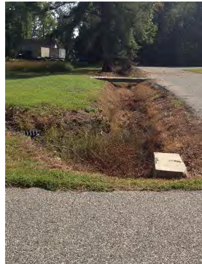
Photo 3 - Peachie Ln. Ditch Looking South
