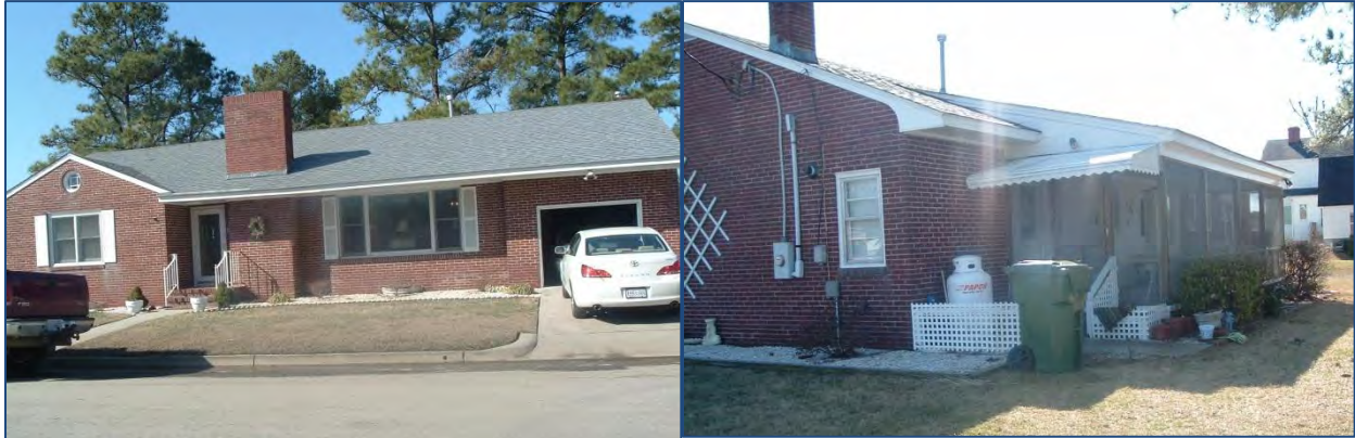
Figure 152: Photos of a home in the Town of West Point before being elevated.
