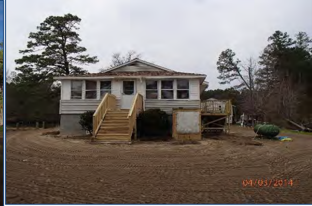
Figure 147: House in Hayes, Gloucester County - AFTER elevation.
