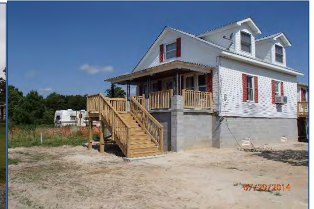
Figure 149: House in Hayes, Gloucester County - AFTER elevation.
