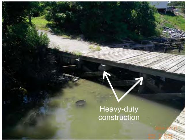
Heavy duty construction consists of 10 in x 10 in cross-beams on the section of pier that is used to load and unload.
