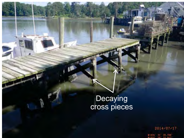
The L section of the docks have X braces that are in various stages of decay.
