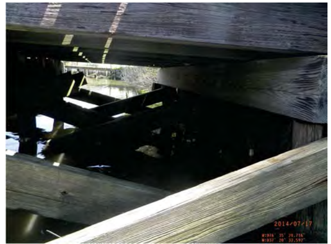
The X braces seem to be intact on the heavy duty section of the dock.
