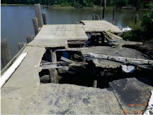
The concrete dock is in complete disrepair and is extremely hazardous. It is presently not in use.
