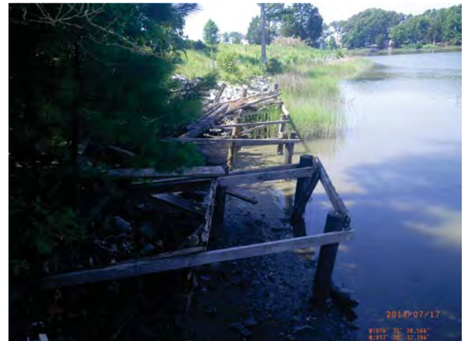
The remains of an old dock could be replaced with a living shoreline to stop the undercutting of the bank.
