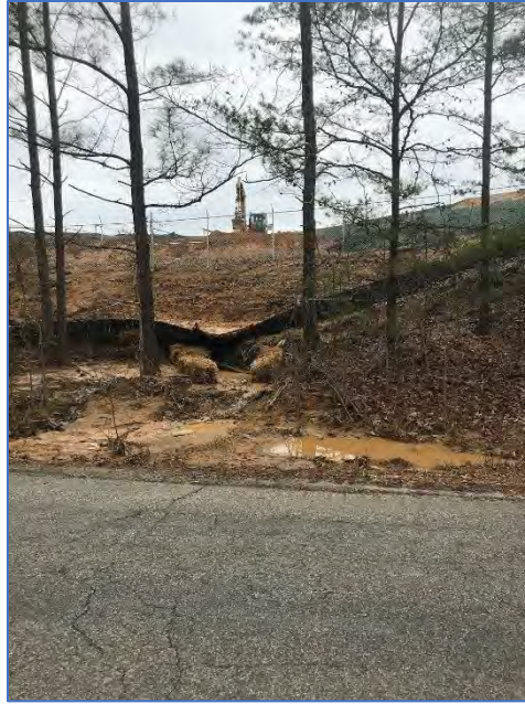
Figure 4: An image of the silt fence being breached at the Essex Solar Center (Friends of the Rappahannock, 2018).
